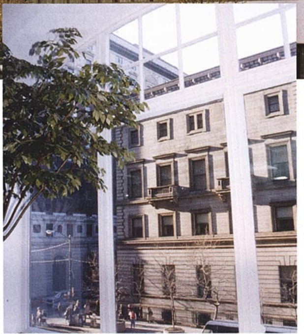
Above: The Hillcrest II in Cincinnati, OH, which utilizes electric heat, had an energy savings payback of 1.9 years with installation of interior magnetic storm windows. Below: The Halle Building in Cleveland, OH, utilizes an interior magnetic storm window with 3/16-inch glass.
